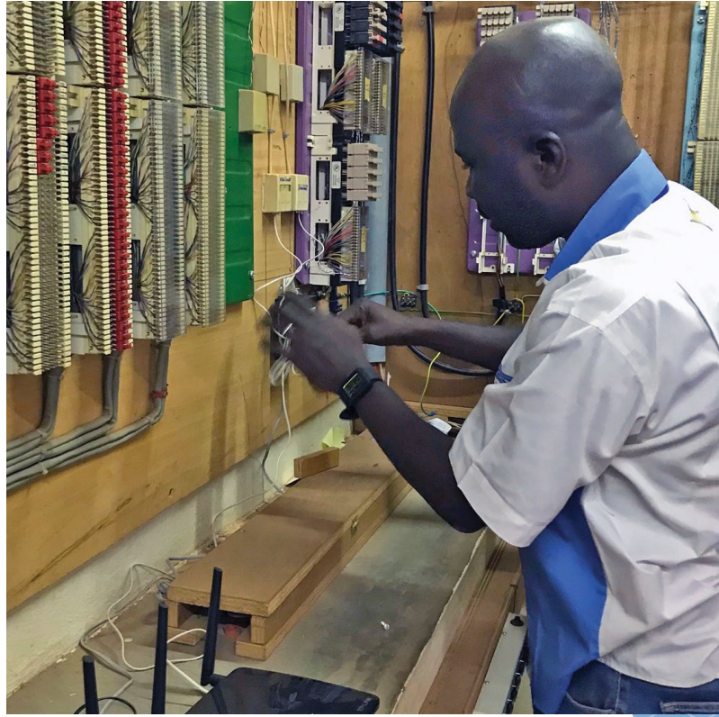
Damien installing the network telephone surge arrester
